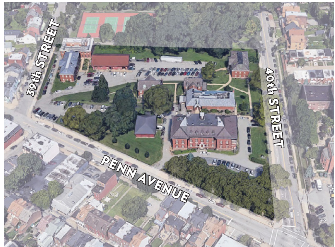
The Clack Campus is bounded by busy roadways: Penn Avenue, 39th and 40th Streets. Arsenal Park forms the Campus' northern border, but the parcels are currently separated by a fence.
