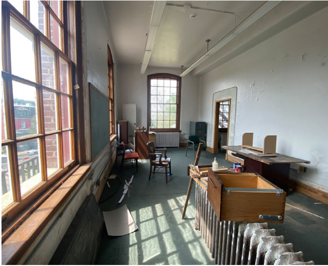
Interior of the Marine Hospital Building's light-filled rooms (building #1)
