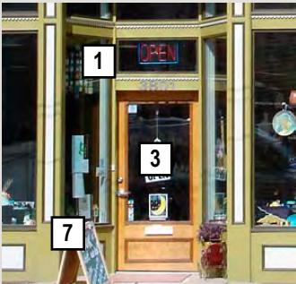
Inadequate latch side clearance
