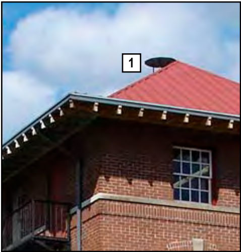
Hip roof with rafter tails on a public building.
