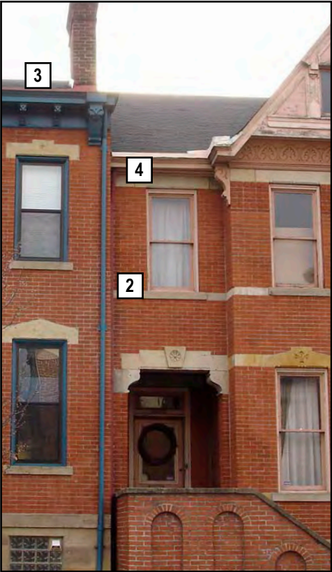
Recessing a residential building's entry provides a layer of privacy from the public street in addition to adding depth and texture to a façade.
