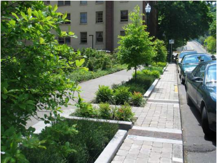
Stormwater can be managed using street infrastructure, before the water enters the sewer system. Additional sidewalk area, tree pits and new curb bumpouts can provide space for integrated stormwater management systems. A stormwater planter in Portland, Oregon.
