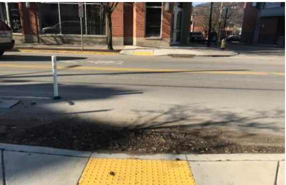
Photo showing an ADA-compliant curb ramp without crosswalk striping in Lower Lawrenceville
