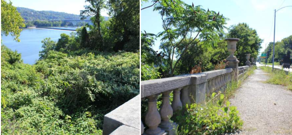
Figures 15 and 16. A view down into the Heth's Run Stream Valley, and the bridge crossing at the edge of Highland Park and Butler Street.
