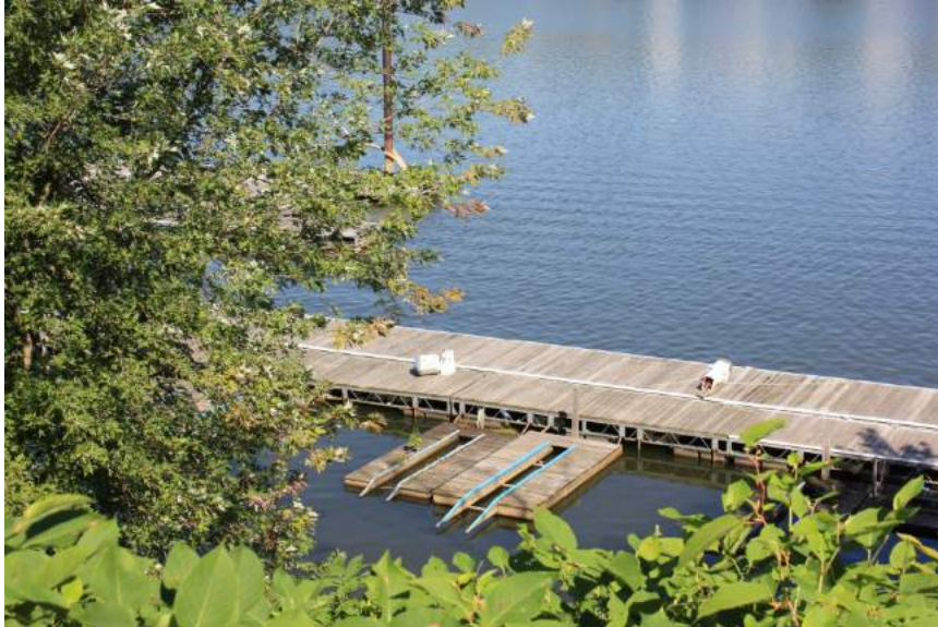
Figure 41. The abandoned marina to the south of the 62nd street bridge crossing provides a unique opportunity for integration of floating wetlands as a public park space.
