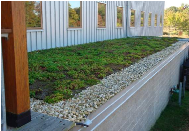
Figure 45. A greenroof provides another layer of habitat and stormwater management, extending the vegetated buffer, even as structures are included on a redevelopment site. © Biohabitats, Inc.
