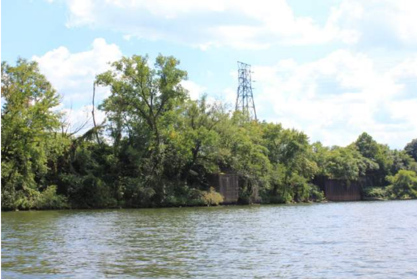
Figure 22. View of bulkhead and riparian edge north and east of 43rd Street.
