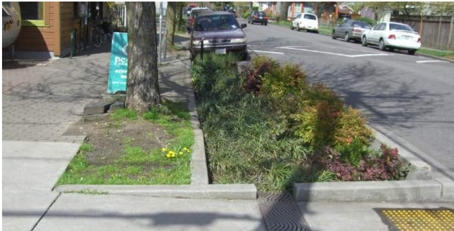
Figure 44. An example of integrated stormwater treatment and native plantings along a streetscape. © Biohabitats, Inc.
