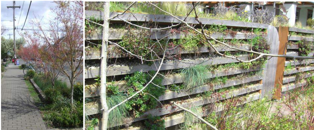
Figures 60 and 61. Streetscape plantings for stormwater management, and vertical plantings for habitat enhancement and stormwater management. © Biohabitats, Inc.
