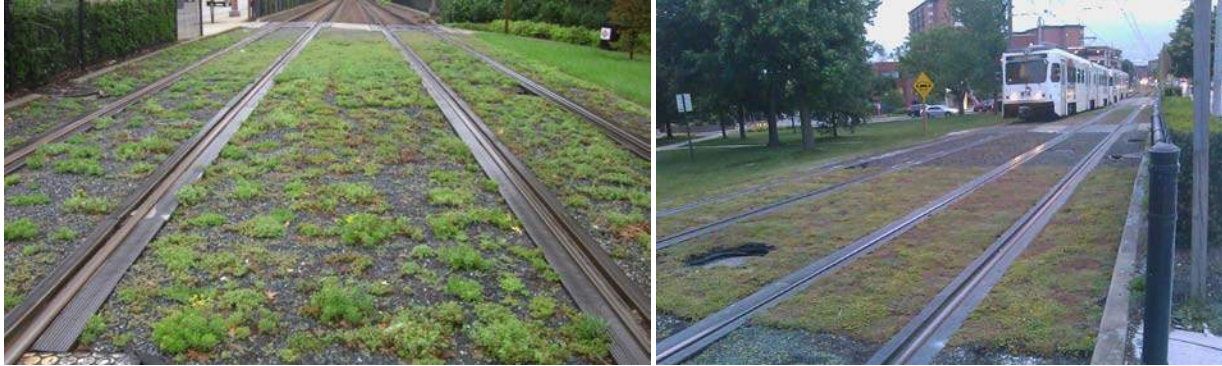
Figures 58 and 59. Planted active rails. © Biohabitats, Inc.
