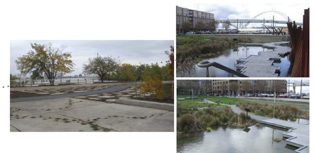
17th Street Wetland and Stormwater Treatment Amenity
