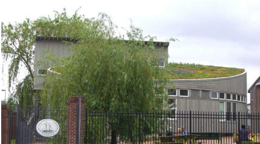
Figures 63. A green roof provides visual amenity integrated into building architecture, stormwater management, and multilayer habitat opportunities. © Biohabitats, Inc.
