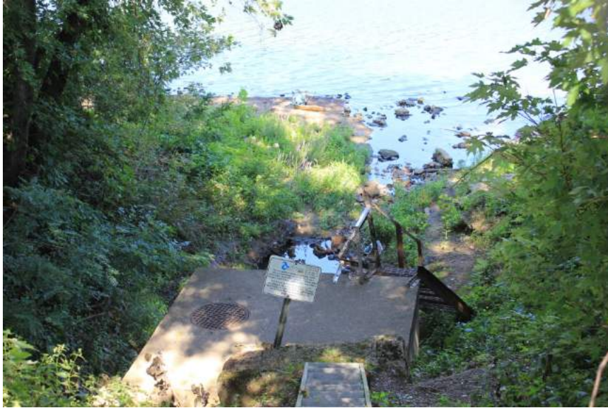
Figure 20. The CSO outfall at 57th Street.
