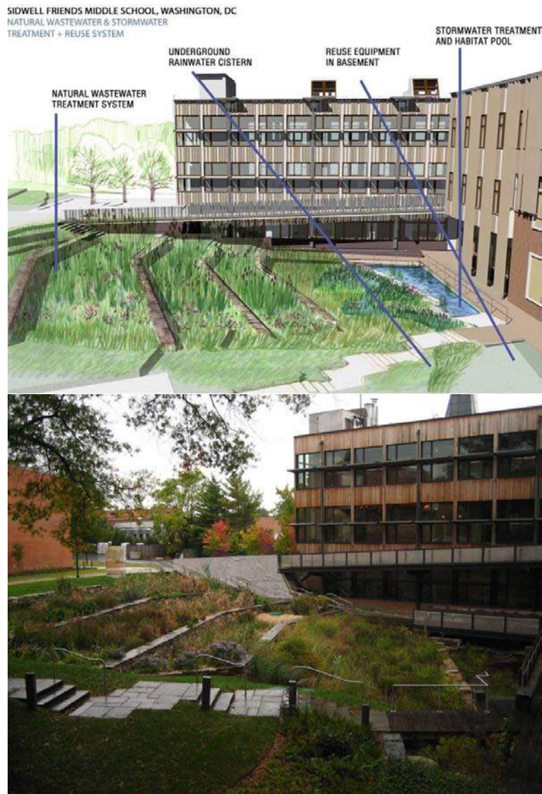
Figures 49 and 50. An integrated wastewater treatment wetland and stormwater amenity integrated into a building's surrounding landscape creates a functional landscape that acts as an amenity, learning space, and treatment zone. Images © Natural Systems International – NSI
