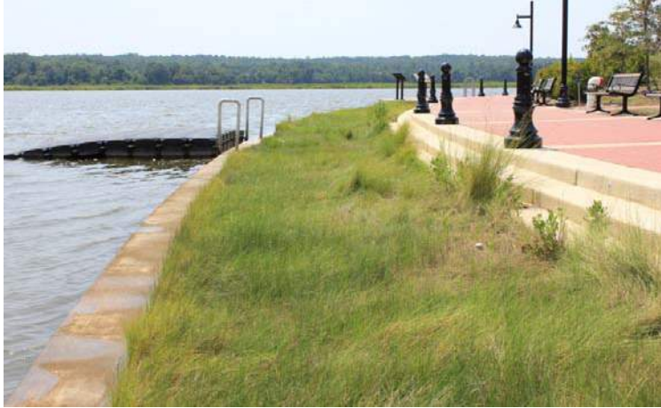
Figure 43. A shoreline treatment where native plantings are integrated into a strengthened bulkhead along a trail amenity. © Biohabitats, Inc.
