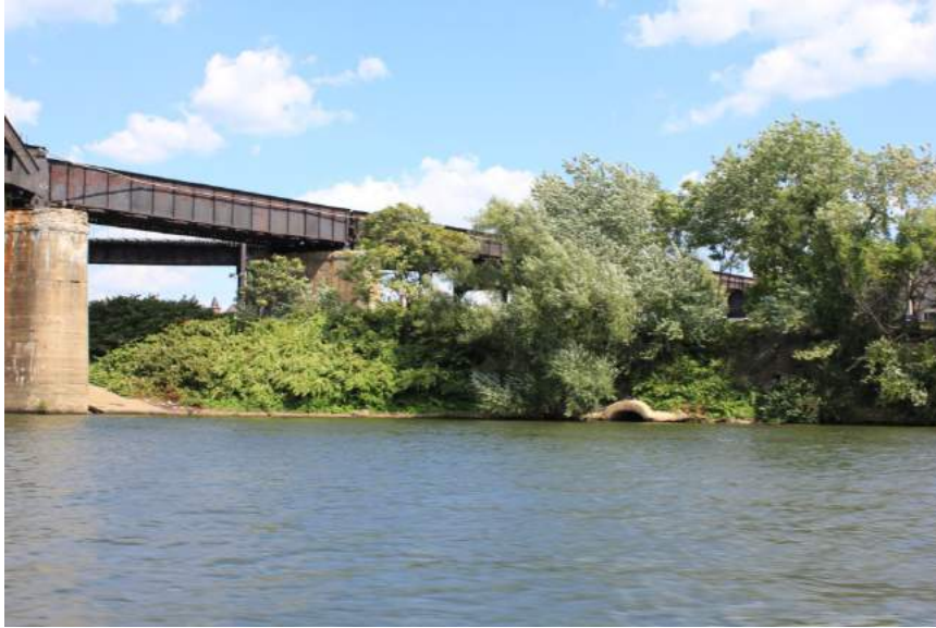
Figure 25. The outfall near 32nd street which may convey flows of the historic Two Mile Run.
