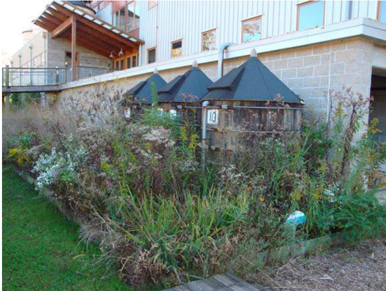
Figure 62. Cisterns and native plantings integrated into structural design. © Biohabitats, Inc.
