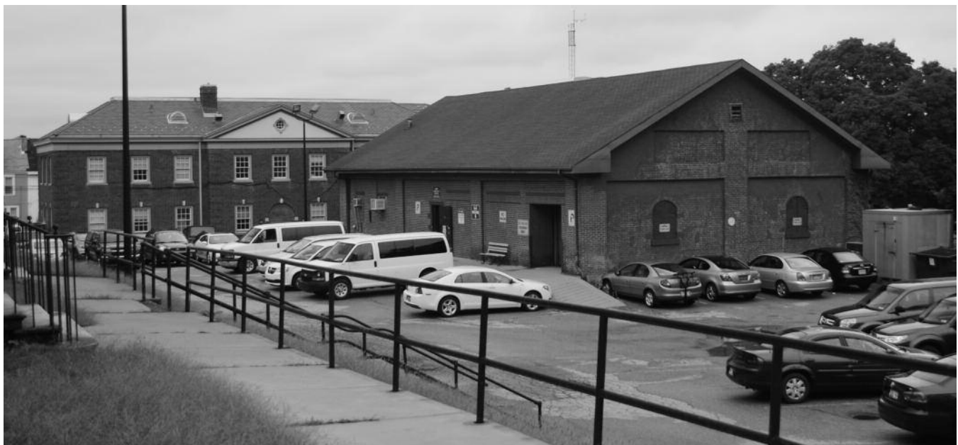
At right is Building No. 6, a former gunpowder magazine, now used as office space. Behind it is Building No. 7, one of four buildings added to the Marine Hospital in 1933. It now houses the county's Air Quality Program.
